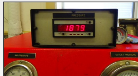
Hose failure at 1879 psi. (exceeding 4:1 safety factor)
